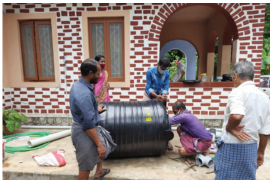
Rainwater filter unit training and installation at Ancham Mile Watershed
