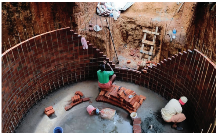
Construction of biogas plant at Kerala Kalamandalam, Cheruthuruthy, Thrissur
