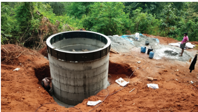
Irrigation tank constructed in Chaliyar Grama Panchayath
