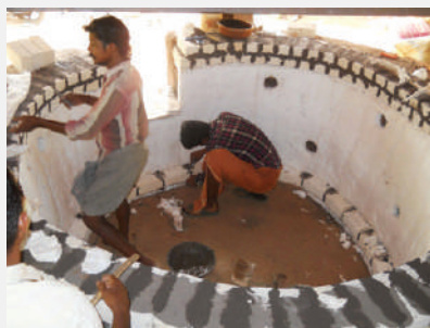
Shri. Vijayakumar supervising the work of insulating the kiln wall with ceramic fibre blanket for better energy efficiency of the Kiln
