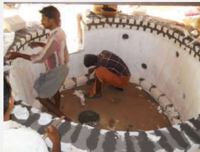
Shri. Vijayakumar supervising the work of insulating the kiln wall with ceramic fibre blanket for better energy efficiency of the Kiln
